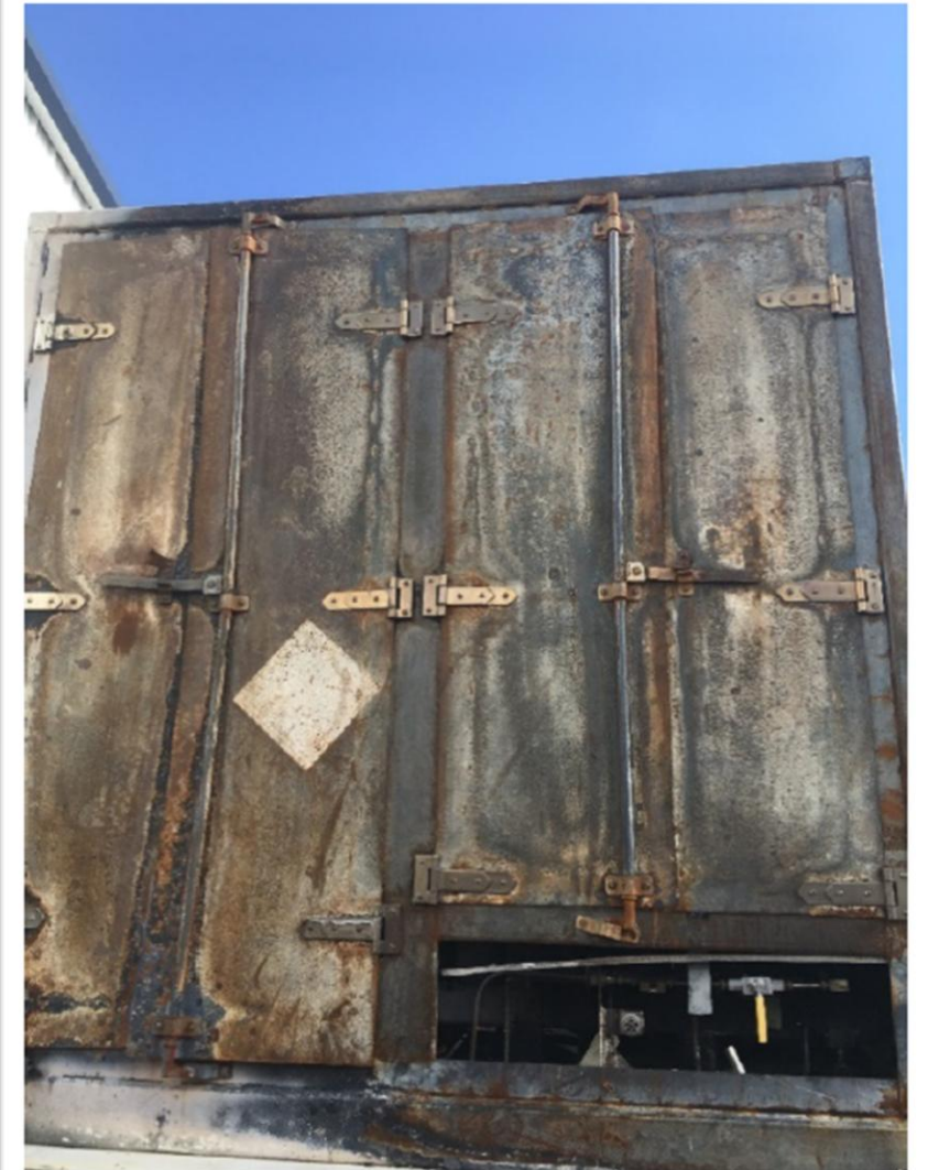
Figure 8. Doors on Rear Module Incident Trailer
